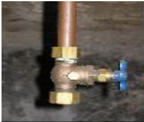
This picture shows brass pipe with fittings containing lead. The lead can leach into drinking water. Run the cold water for few minutes to eliminate most potent lead hazard in the water.
